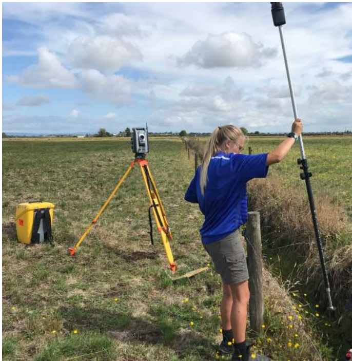
Laser surveying peat and drain levels
